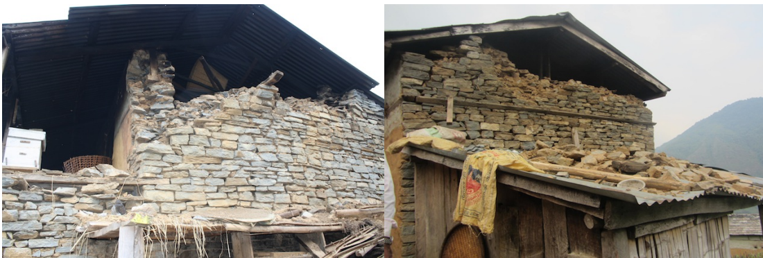
Damaged houses in Khanche village, which got flat later on 12 th May 2015, 7.4 magnitude of earthquake
